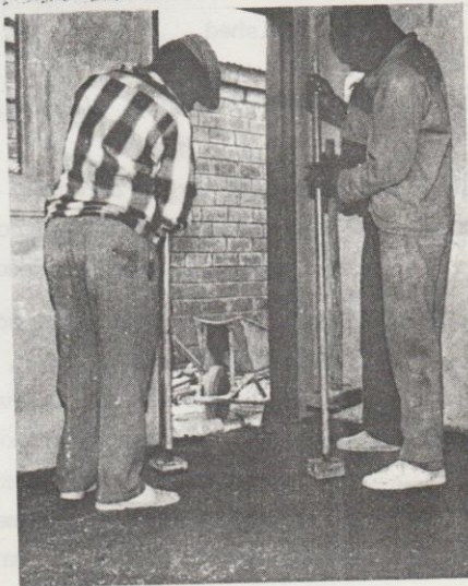
Fig.4.2. COMPACTING THE SUB-FLOOR
