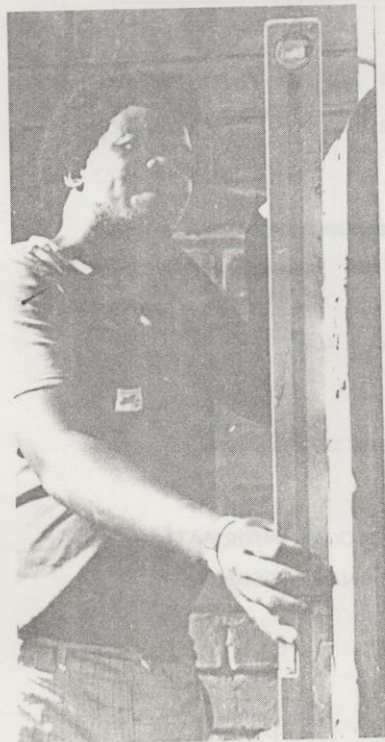
Fig.5.8. LEVELLING VERTICALLY
